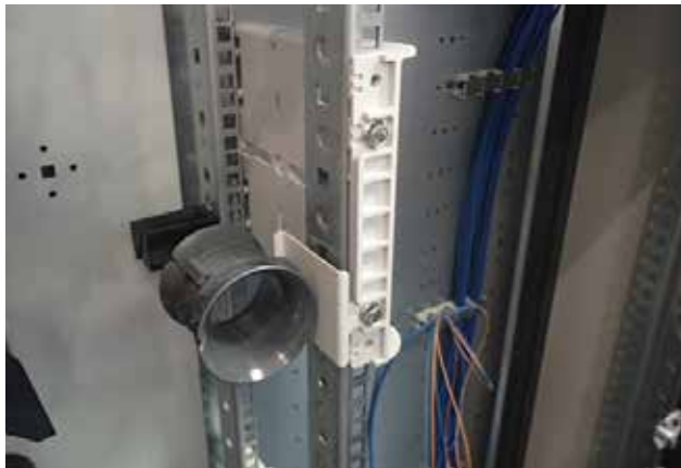
2 Montage du kit bobine (e + j/d) Mounting spool kit (e + j/d)
