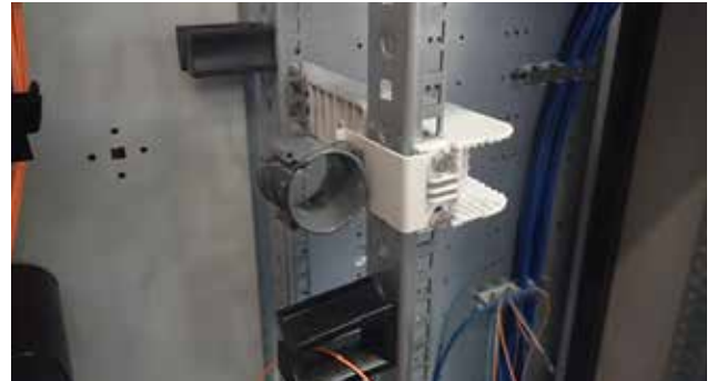
2 Montage du kit bobine sans plaque (e + d/l) Mounting spool kit without plate (e + d/l)
