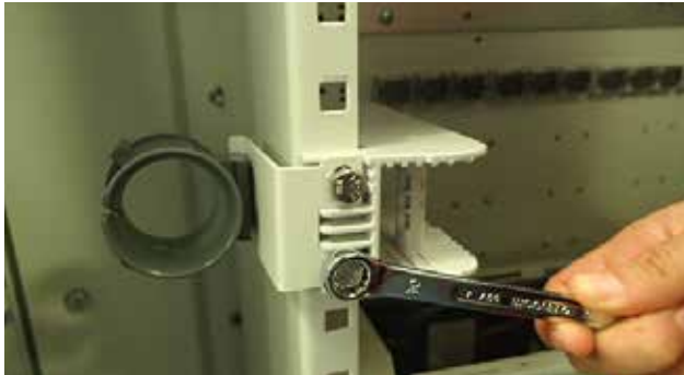
2 Montage du kit bobine sans plaque (d + e) Mounting spool kit without plate (d + e)
