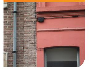
This cable has a capacity from 24 to 96 fibres. Access to the fibres by window cut is quick and easy thanks to a flexible UV resistant sheathing material. Each units can be pulled back on more than 1m to easily connect the facade distribution box.
